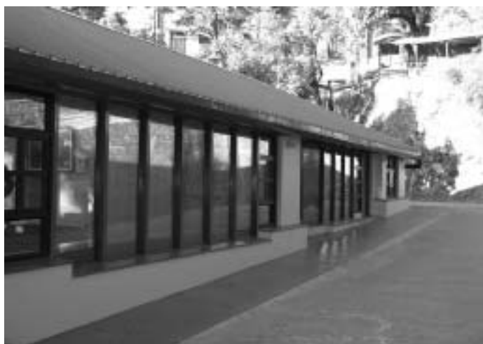
After: The newly refurbished Business Center
